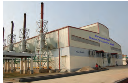
51 MW rental power plant of Barakatullah Electro Dynamics Ltd.
