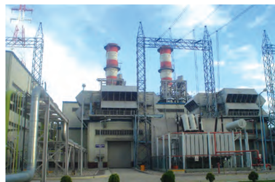
450 MW Meghnaghat power plant
