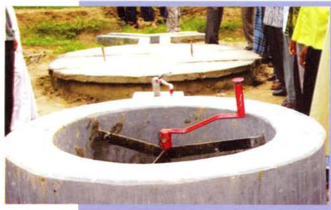
A biogas plant financed by IDCOL
