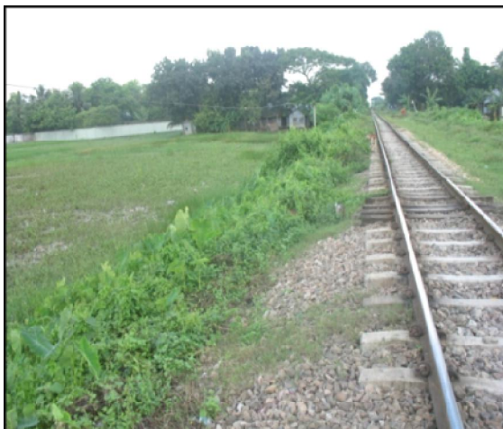
Photo 3.6: Rail way crossing beside the power plant
