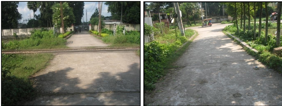
Photo 3.1: Approved and existing Access Road from Comilla-Laksham highway to the PGCB Substation
