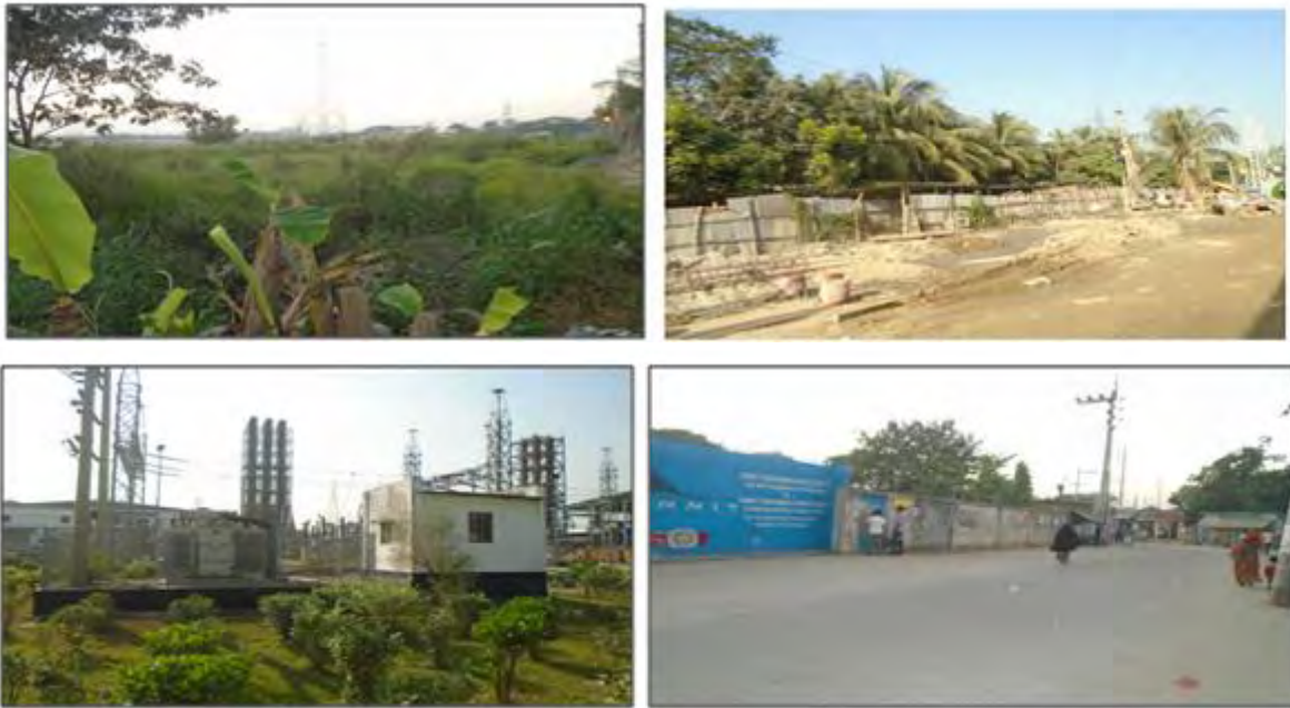
Photo 7.1: Site view for the main plant SNPL UNIT II Unit II
