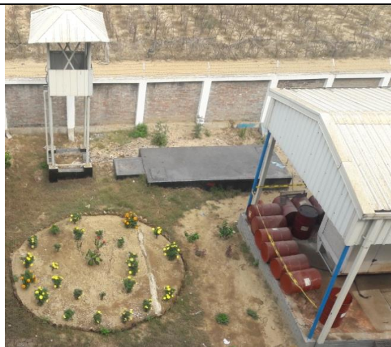
Photograph: Garden near generator
