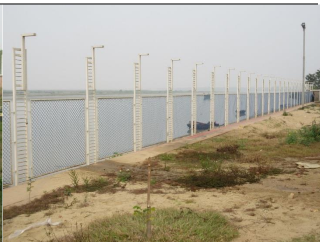
Photograph: Fencing wall at river side
