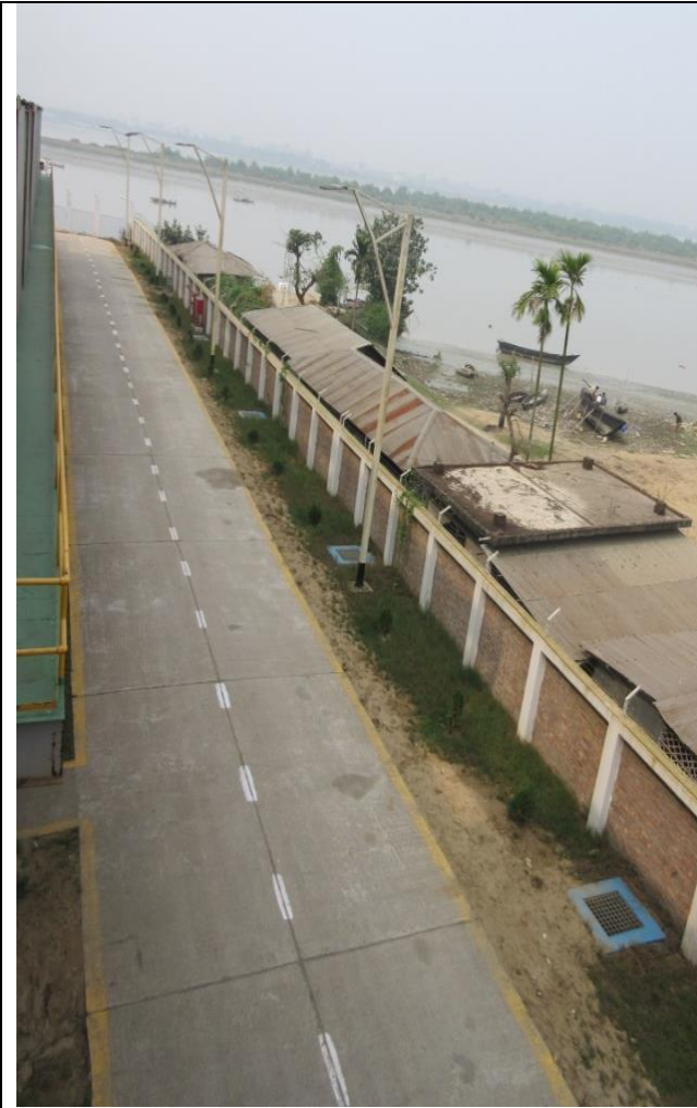
Photograph: External housekeeping
