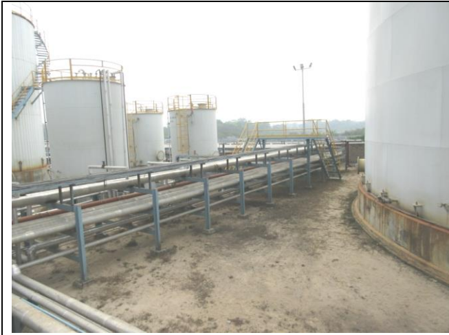
Photograph: Safety bund around fuel storage tanks
