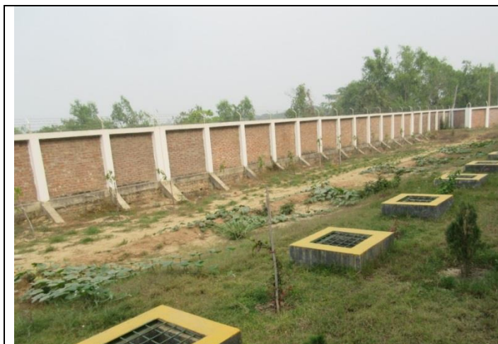
Photograph: Brick wall around village side
