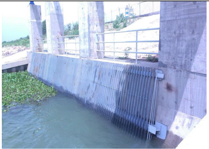
Photographs: Thermal balancing drainage and screen at outlet
