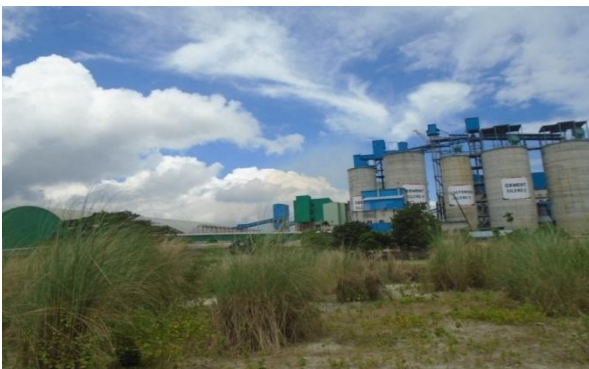
Photo 6.7: West side for alternative site 2
