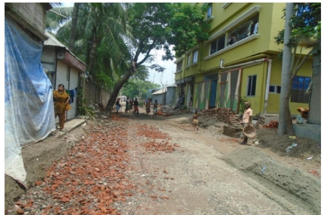
Photo 3.3 : 6.3 m wide and 750m long access road from the project site to district main road are constructing by the SAPLRT authority
