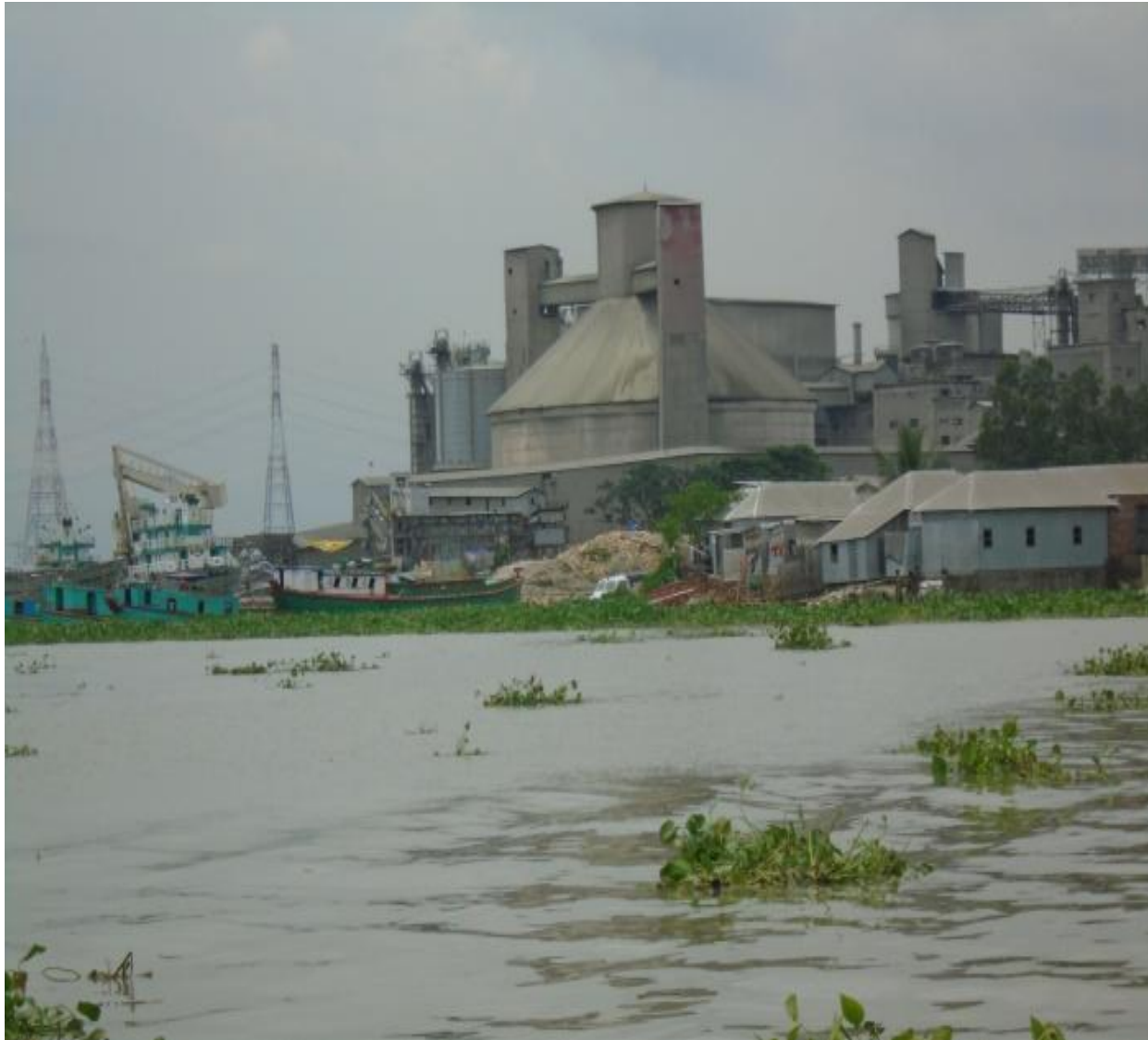
Photo 3.6: Crown Cement factory adjacent to the project site
