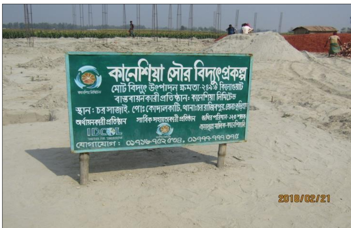
Figure 3.3: Sand Filling Activities in the Project Area
