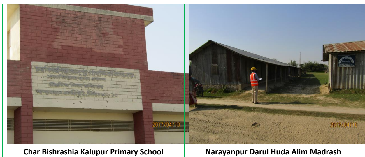
Figure 8.15: Physical Resources in the Project Area
