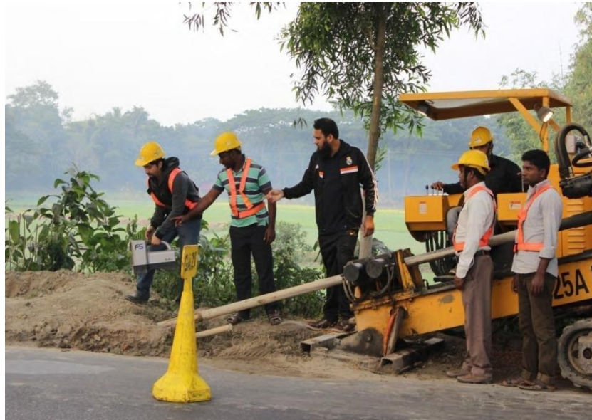
Figure 3.2: Horizontal Directional Drilling (HDD) Machine
