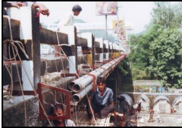
Figure 3.6: Bridge crossing of fiber optic cable using DWCC Pipe with Clamping.
