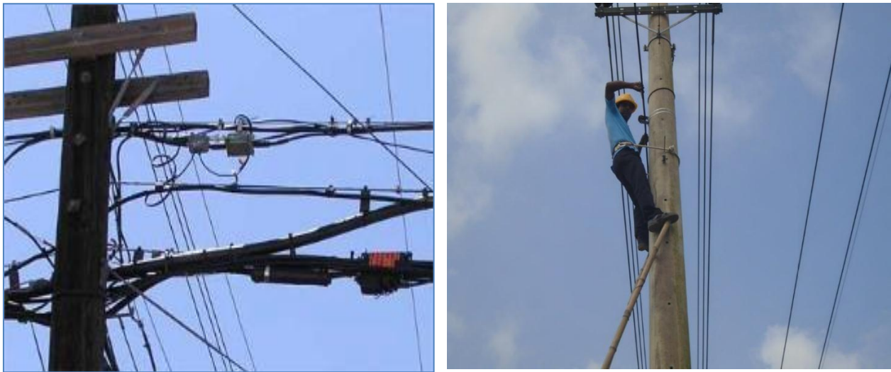
Figure 3.8: Installation of overhead fiber optic cableline.
