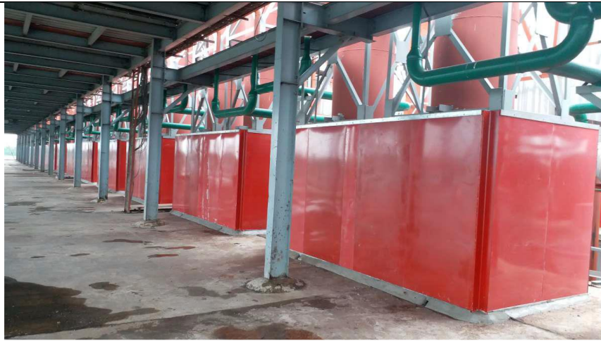
Photograph: Acoustic box surrounding exhaust fan of engines
