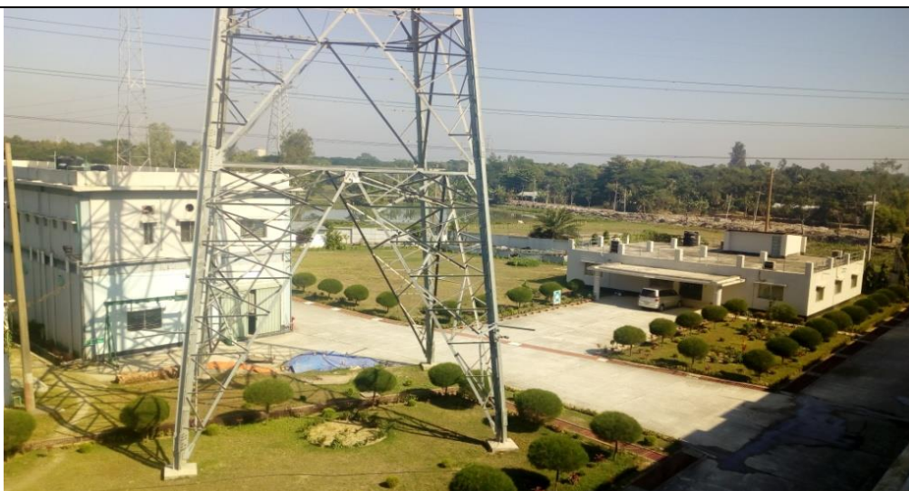
Photograph: An external view of administrative building and dormitory
