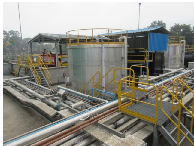
Photograph: Safety bund around fuel storage tanks
