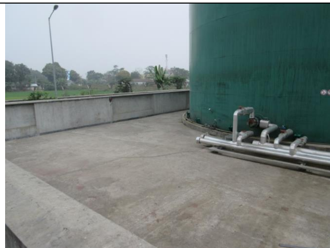
Photograph: Safety bund around fuel storage tanks
