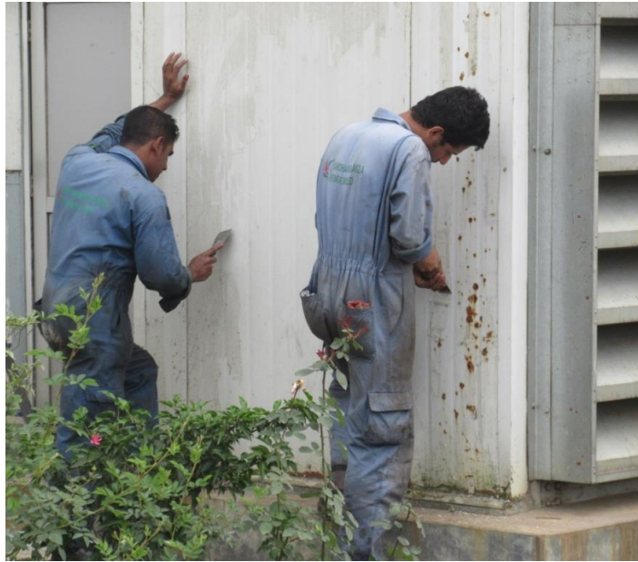
Photograph: Arrangement of PPE
