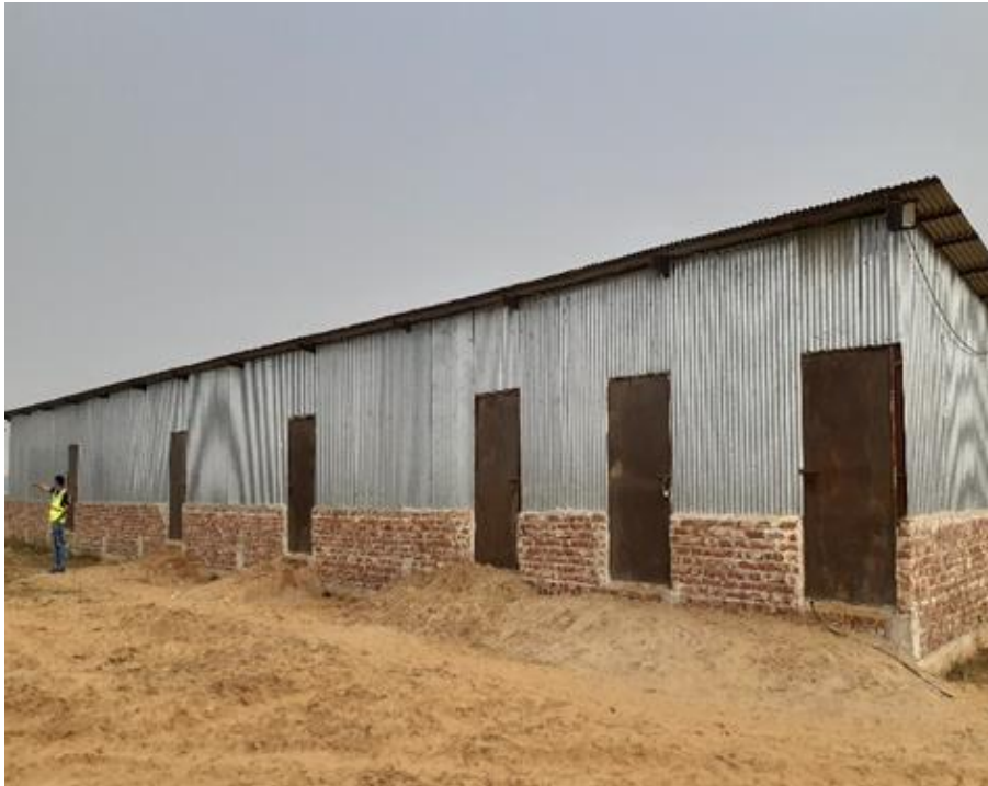
Photograph 9 (a): Accommodation for Workers
