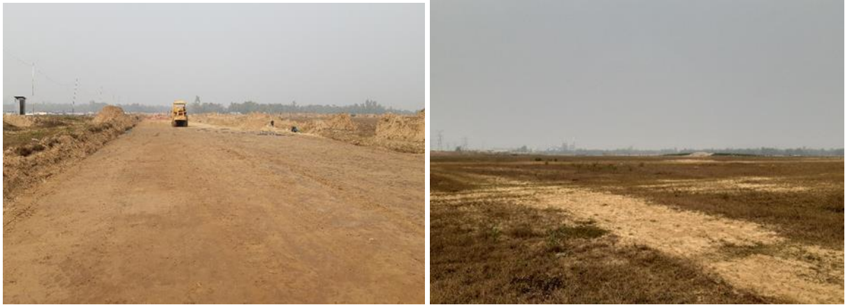
Photograph 8: Current status of the site
