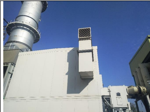
Photograph: Acoustic box surrounding exhaust fan of engines
