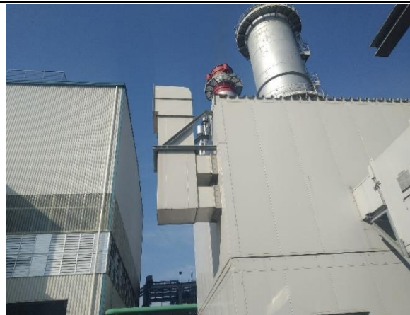
Photograph: Acoustic box surrounding exhaust fan of engines
