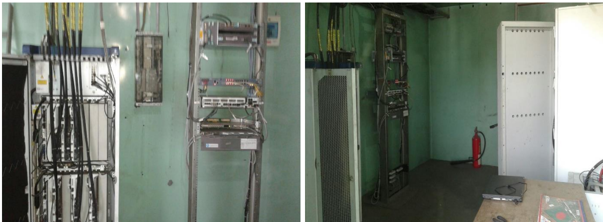
Figure 3.7: Indoor picture of tower station
