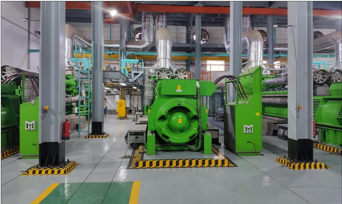
Figure 3-3: Power generating Engine
