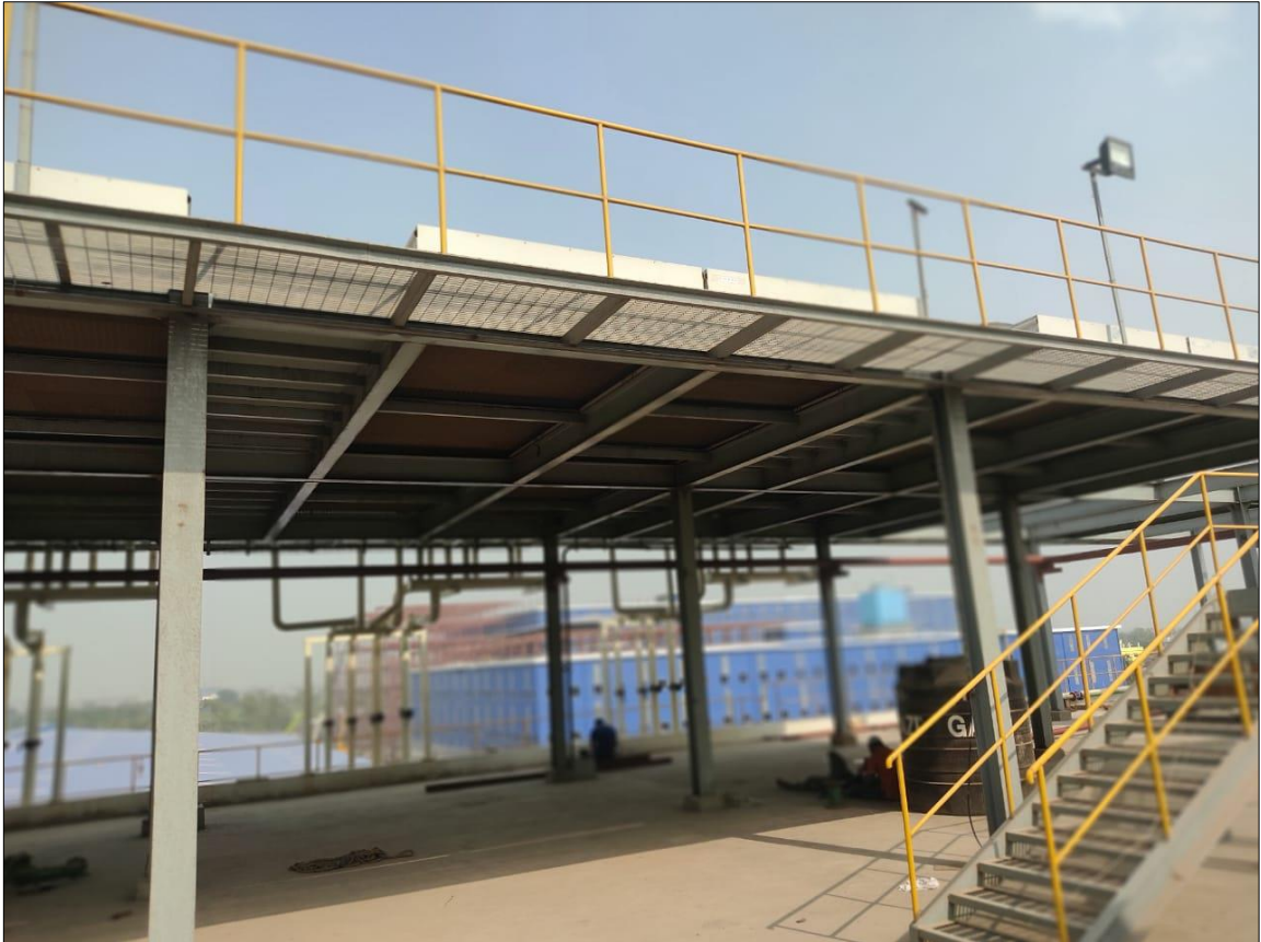
Figure 3-7: Water Cooling tower.
