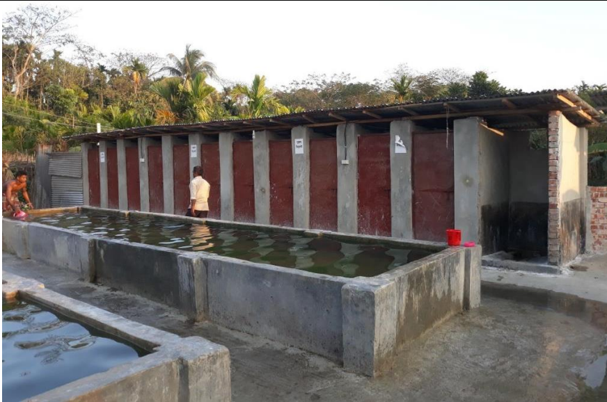
Photograph: Toilet and cleaning facilities
