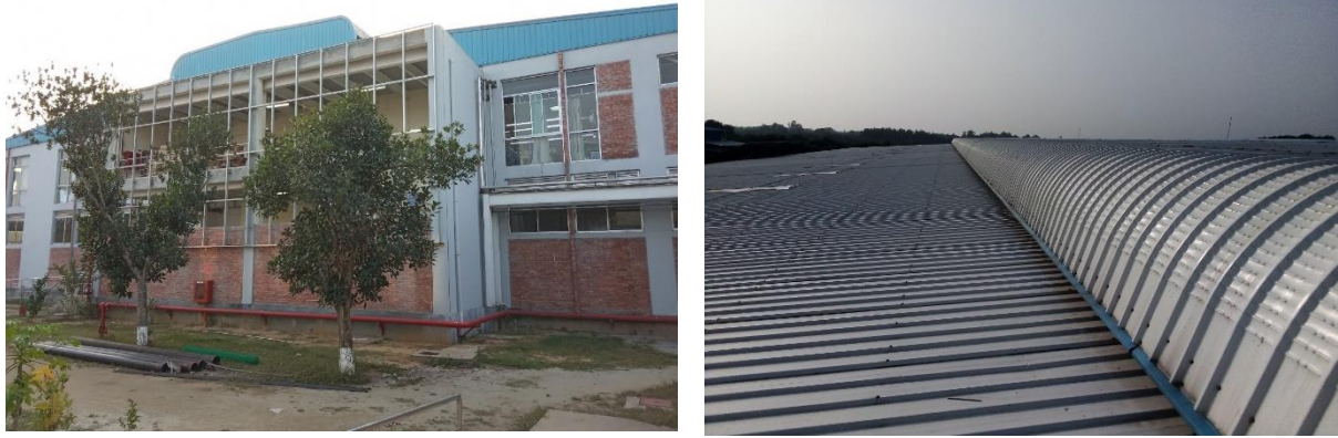
Figure: Photos of the main building and the rooftop
