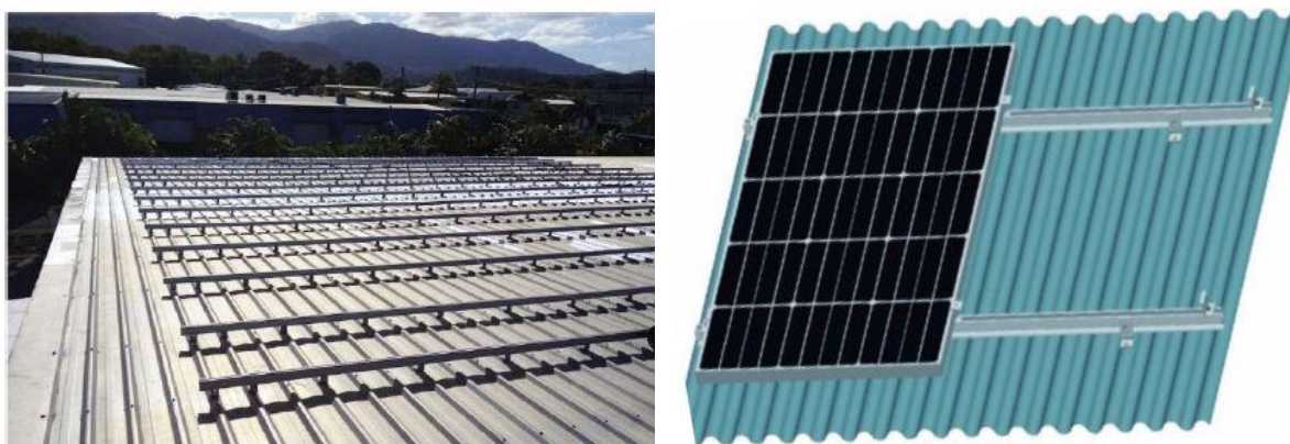
Figure 3.5: Metal Roof Mounting Structure
